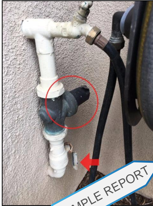
Shut off lever and gas regulator
