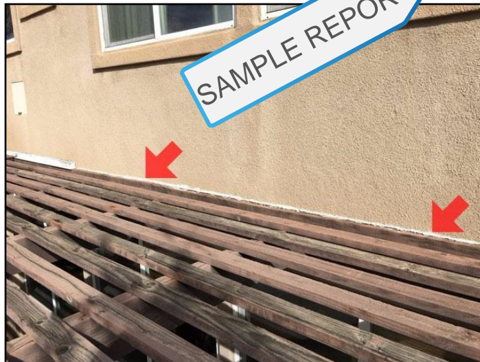
Missing flashing
