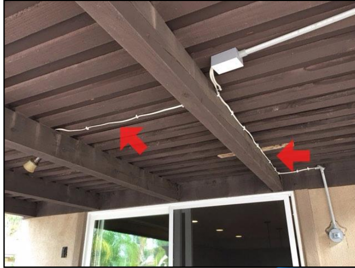
Exposed wires
